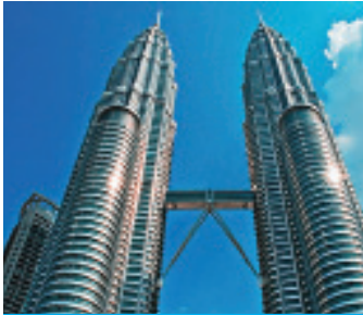
Petronas Twin Towers
